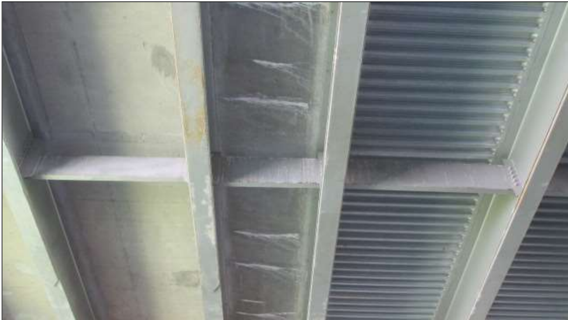
BAYS 4, 8, AND 12 ARE CLOSURE POURS BETWEEN THE ORIGINAL AND NEW SECTIONS OF THE BRIDGE. THESE BAYS HAVE HAIRLINE TRANSVERSE CRACKS WITH EFFLORESCENC
