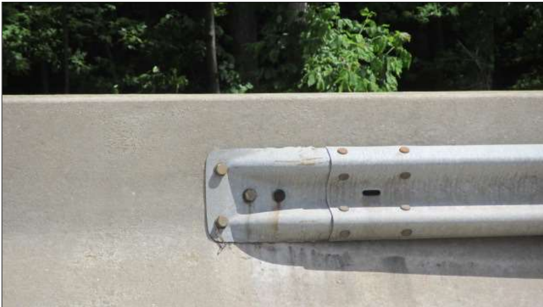
GUARDRAIL ATTACHED TO THE BRIDGE RAIL FOR ALL FOUR CORNERS
