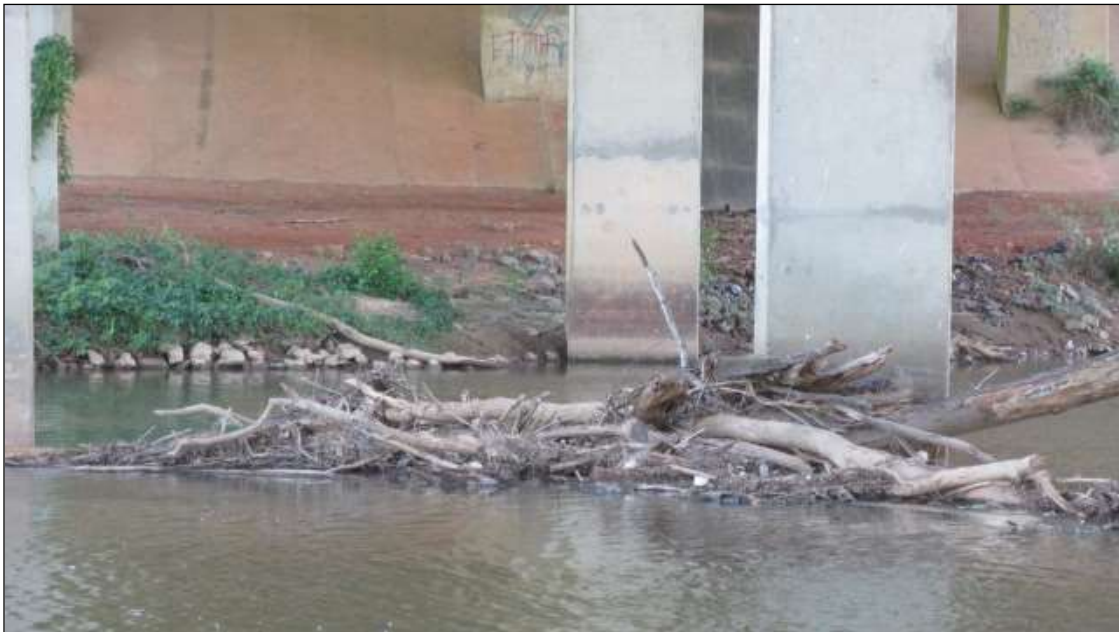
DRIFT ALONG BENT 10 5' WIDE X 12' LONG AT BENT 10
