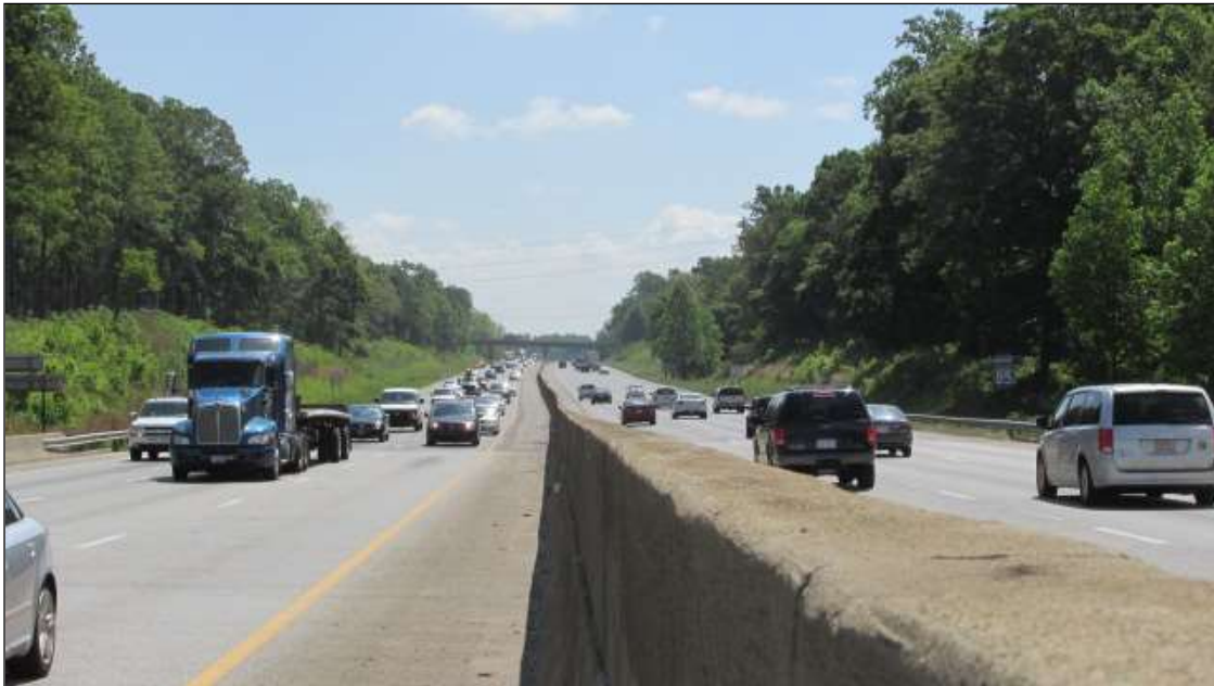
GUARDRAIL LOOKING NORTH
