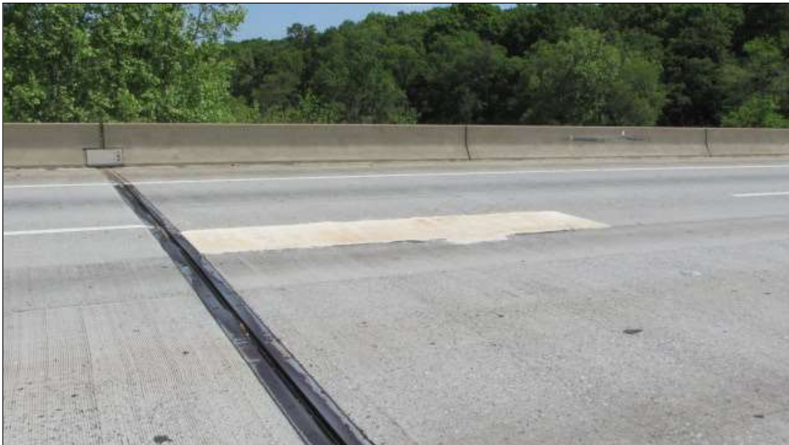
THERE IS SCAT. LARGE CONCRETE PATCHING IN ALL SPANS OF THE NBL ESPEC. ALONG THE CENTER LANE.
