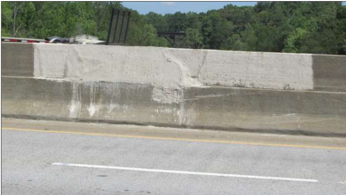
20' SWCTION OF CONCRETE RAIL REPAIRED OVER BENT 5.
