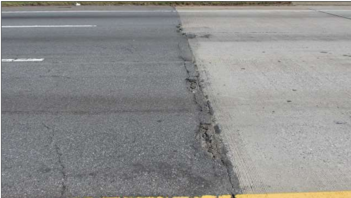
THE SOUTH APPROACH ALONG THE NORTH BOUND LANES HAS CRACKING ALONG THE END SPAN.
