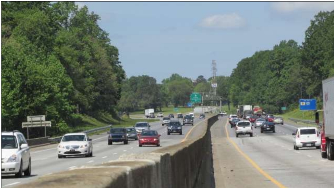
GUARDRAIL LOOKING SOUTH
