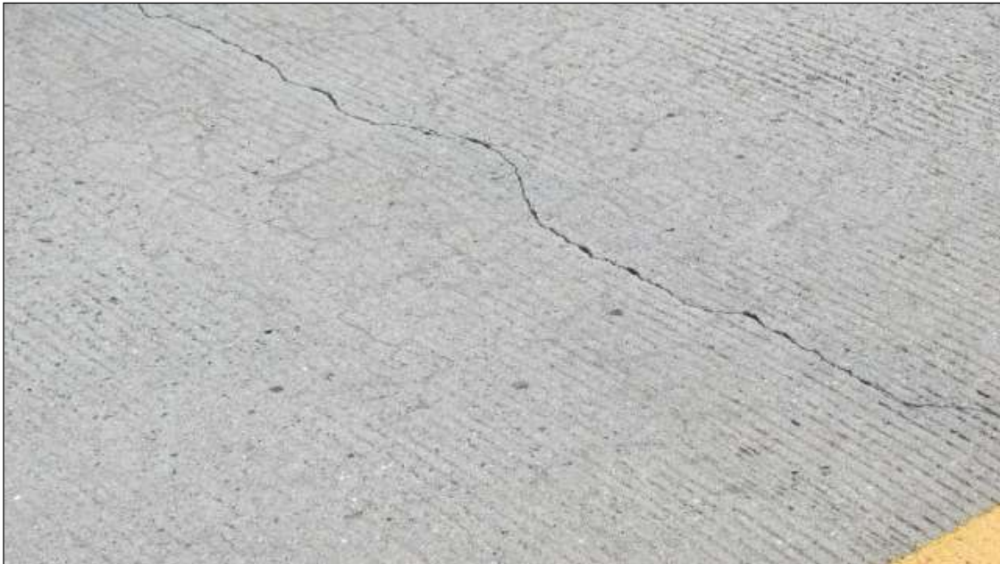
TRANS. CRACKING PRESENT IN SCAT. AREAS OF ALL SPANS.
