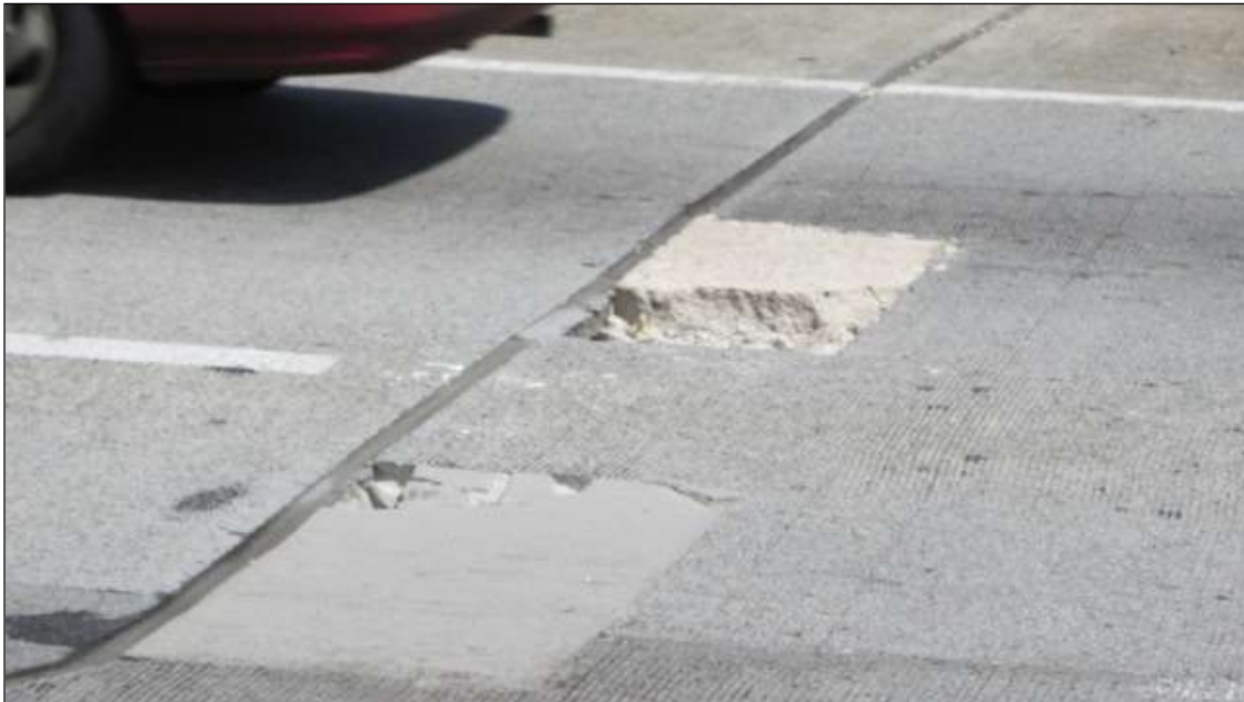
LARGE CONCRETE PATCHING ALONG BENT 2 IN THE NBL.
