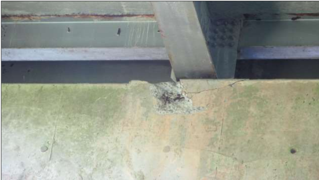
THERE IS A 32"LONG X 13" H X 2 1/2" DEEP ON THE SOUTH FACE OF BT.8 UNDER BEAM 2 W/ REBAR EXPOSED.
