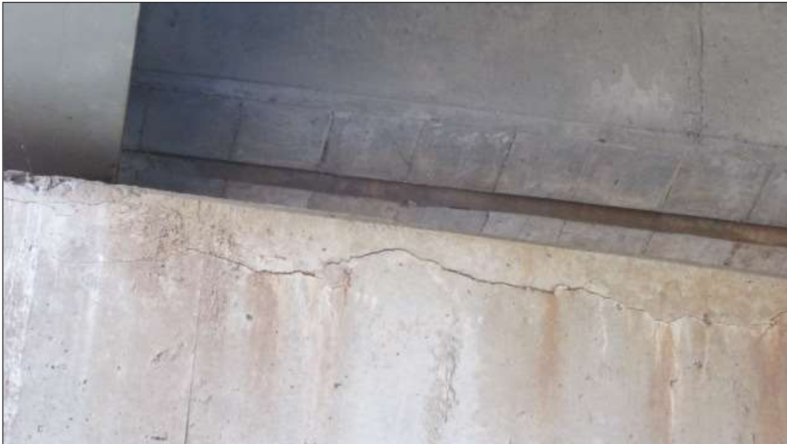
HORIZ. CRACKING ALONG THE THE NORTH FACE OF BENT 2 IN BAY 2 AND 3 ALONG THE TOP. FOR 6' TO 8'
