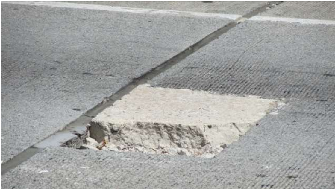
BENT 2 CONCRETE PATCH IN THE CENTER LANE 2' WIDE X 3'4" LONG. THE PATCH IS ALONG THE JOINT. AND BREAKING OUT 1' WIDE X 3.5 LONG. IN THE NBL SPAN 3. CE
