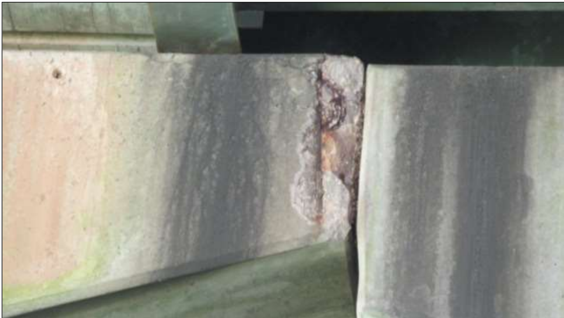
THERE IS A SPALL 3" WIDE X 18" WITH REBAR EXPOSED.
