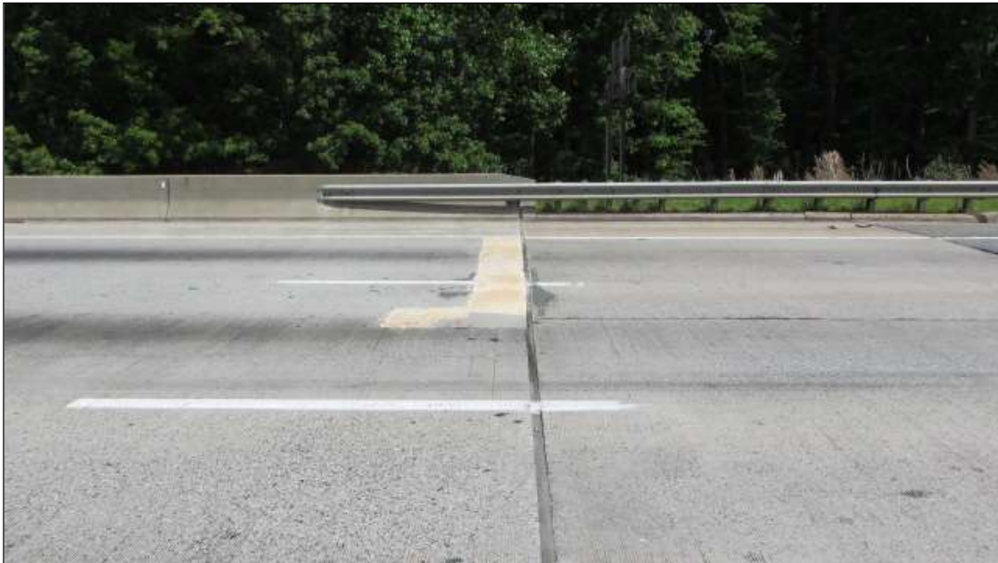
CONCRETE PATCHING ALONG THE END SPAN AND THE NORTH APPROACH IN THE NBL.
